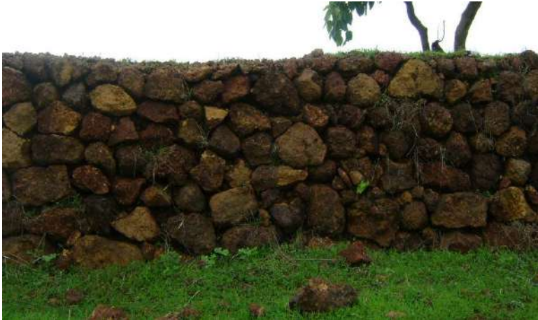
Retaining wall for control of erosion during monsoon season.
