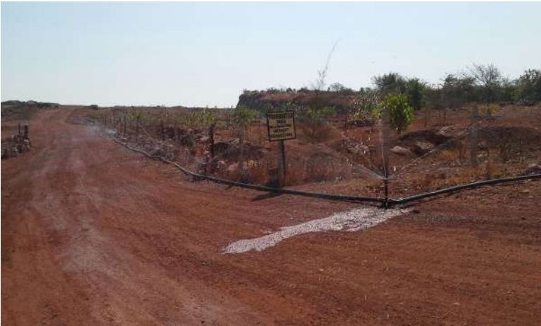
Dust Suppression System on Haulage Road at Mines
