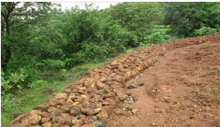
Retaining wall made for control of erosion.
