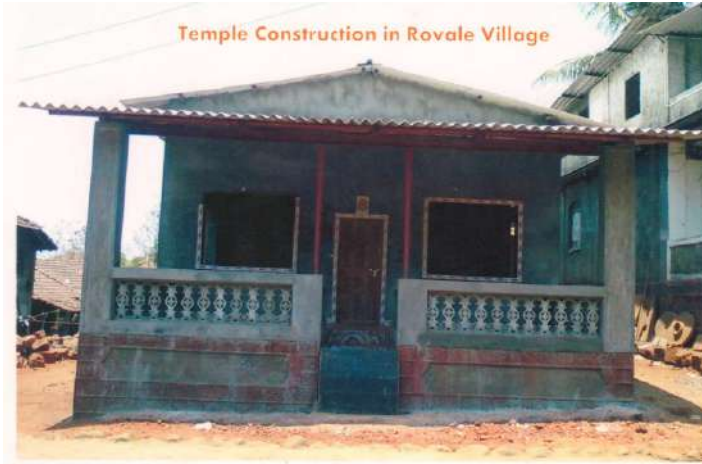
Temple Construction at Rowale Village
