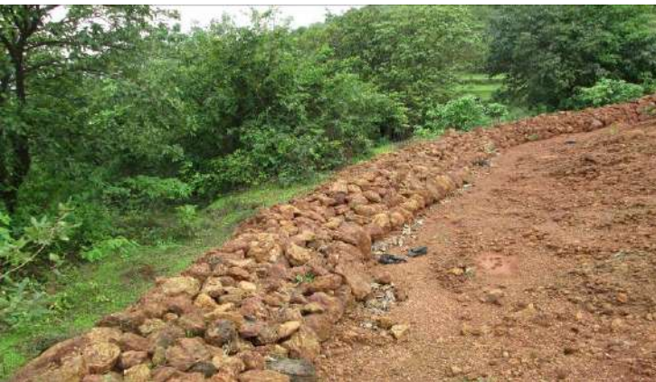
Retaining wall made for control of erosion.
